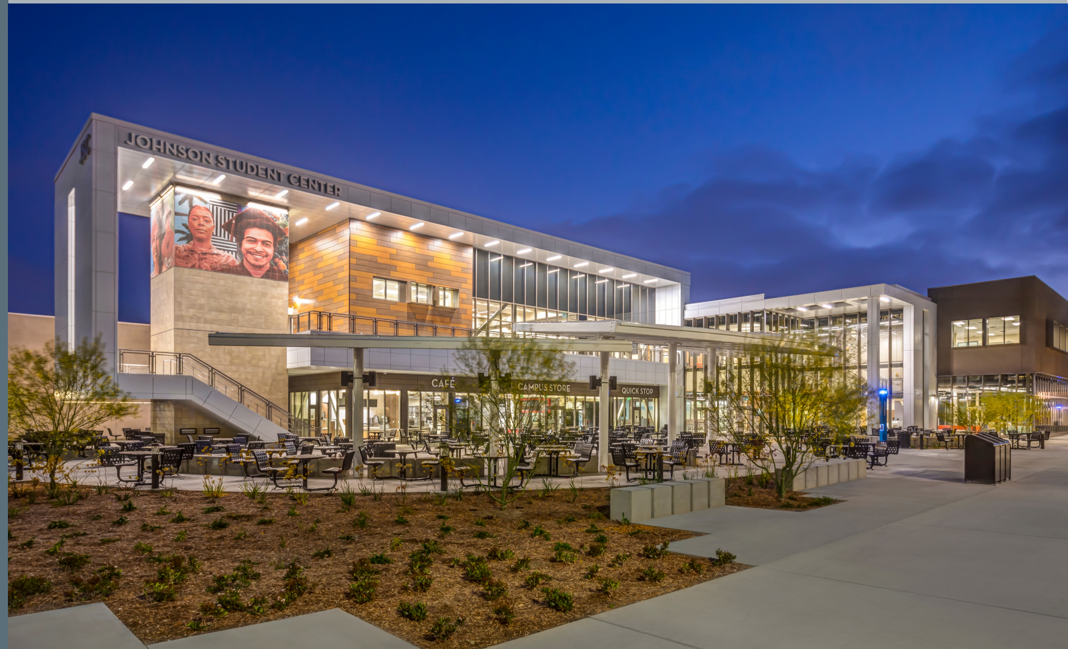
Photo: Santa Ana College Johnson Center, Santa Ana, CA Designed to meet LEED Silver Certification
